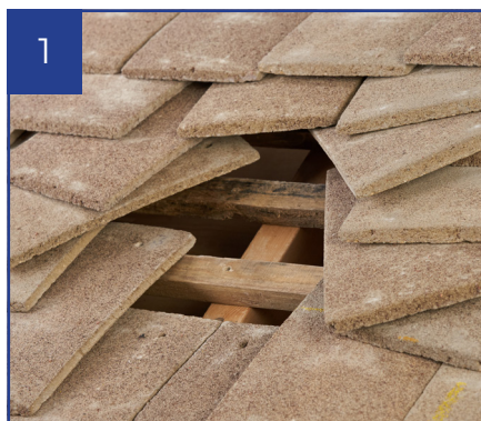
Remove tiles to reveal rafter.
