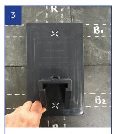
Place Limpet in the fixing position shown to spread any compression load to the battens B1 & B2. Drill through each X marked fixing point on the Limpet using a 7mm tile drill. Sufficient to mark the slate below.
