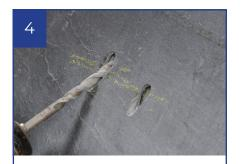
Drill out the two marked holes through the slates being careful to avoid penetrating the underfelt. Once through the slates, continue drilling bringing the drill slowly down from vertical to horizontal, thereby elongating the two holes.
