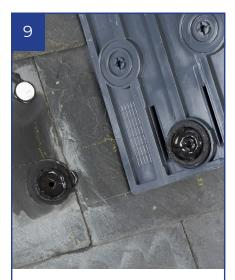
**FOR ILLUSTRATIVE PURPOSES** Image shows how CT1 sealant has been distributed within the EPDM seal once fitted.
