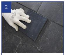
For this application, the limpet base plate buts up to the slates lap. Positioned between two rafters and about 250mm below the internal loft underfelt lap.
