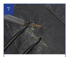
Remove the baseplate section, and drill through the slate with the 1/8th of an inch drill bit. Self tap a small wood screw through the hole and then remove.
