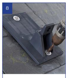
Fix into place using the screws & aluminium EPDM washers supplied. Tighten only until the aluminium washer cover starts deflecting.
