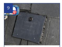
Place the limpet base plate section over the cables. Insert and tighten the wood screw to secure it. Apply CT1 sealant around the top and sides of the base plate, screwhead and slate abutments above the base plate.
