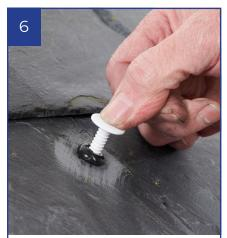
Apply a small blob of CT1 onto the test hole & insert the white plug to seal. Ensure the slate surface is clean and dry. **DO NOT APPLY IN THE RAIN**
