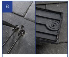
Clean and apply CT1 sealant around the cable entry points, and the drilled hole. Apply CT1 sealant to the top and side edges of the limpet base plate section.
