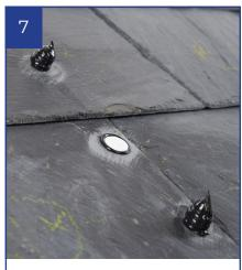
Apply CT1 onto each fixing hole, leaving a 20mm diameter raised portion over each point.
