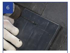
Place the baseplate over the cables, butted up to the slate lap. Using a small 1/8th of an inch drill bit, drill through the dimpled top fixing point of the baseplate just far enough to mark the slate surface.
