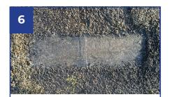
Or you may have to clear a larger area such as on asphalt type roofs with stone chippings and or a lot of moss growth etc. Ensure the area is made reasonably smooth and dry before proceeding.
