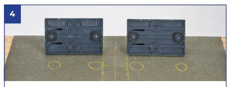
Lift both limpets and note/mark the general seal fixing areas. If you have opted for 4 fixings also note/mark the optional side fixing areas as well. These areas must be clean, reasonably smooth and dry before attempting to fix the Limpet to the roof.
