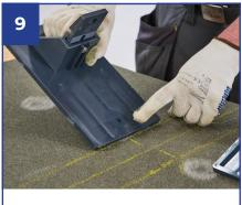
Realign both Limpets into the positions previously marked in step 3.
