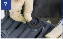
Ensure the EPDM seals have been fitted to the 2 or optionally 4 fixing points. If you are opting to use 4 seals, additional seals, fixing screws, and washers will be required.
