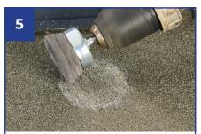
You may be able to simply wipe and dry the roof surface and or lightly buff the surface with a rotary wire brush to clean and dry each fixing point.
