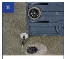
Applied correctly, the CT1 sealant will fill the inner seal housing and screw penetration as illustrated.
