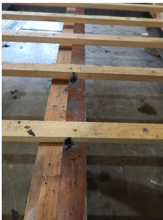
Figure 19 Image to highlight the CT1 sealant on the rafters after testing.
