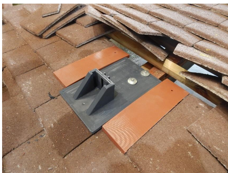
Figure 8 Fixing option 2 using blanking plates in the installation of the PV bracket.
